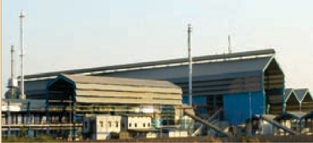
Plant at Samakhiali, Kutch
